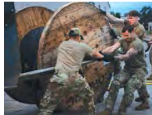
U.S. Air Force Airmen assigned to Ramstein Air Base, Germany, set up an electrical system at Ramstein Air Base, Germany, Aug. 19, 2021.
